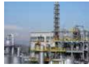
Sulphur-based chemicals Production Plant ITALY
